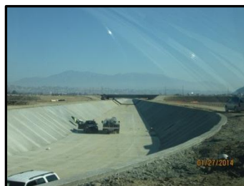
Looking east upstream from the Channel Outlet.
