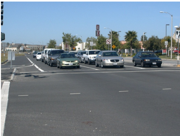
Pictured above are the two existing eastbound lanes of Cactus Avenue which will be widened to add a third lane to increase the level of service during peak traffic congestion times.
